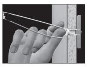
Place thumb between straps at wall. Push thumb side to side, snapping off straps level with flange of cap.
