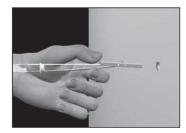
Drill 1/2" hole. Hold metal channel flat alongside plastic straps and slide channel through the hole. Minimum clearance behind wall is 1-7/8"
