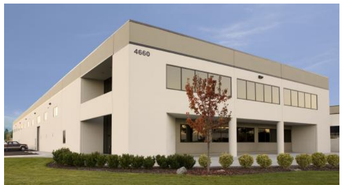
Grumman Building: Assembly and Shipping
